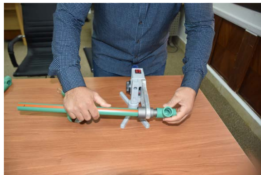
3. Pipe and fitting have to be heated simultaneously. Push in parts to be joined axially.
